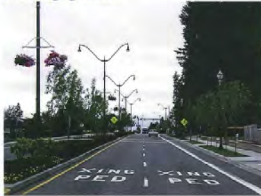
Lighting on Planted Median with Hanging Baskets
