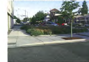
Stormwater Rain Garden
