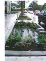
Stormwater Treatment Area in Action
