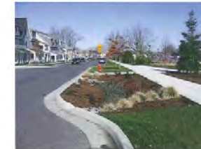
Stormwater Planting Area in Curb Extension
