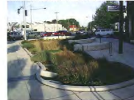
Stormwater Rain Garden
