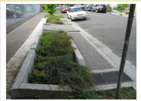
Bioretention planter in the landscape strip manages stormwater runoff in the ROW. See below for standard engineering plan for a similar facility. (Photo courtesy Muralmouth.Wordpress)
