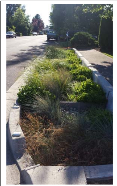
An example of a bioretention area built to capture street runoff. (Photo by Otak, Inc.)
