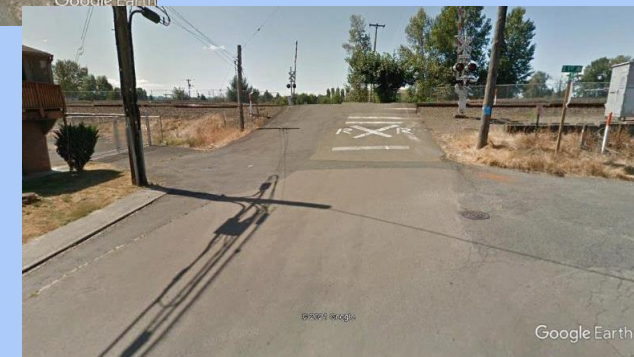
Existing Mill Street
