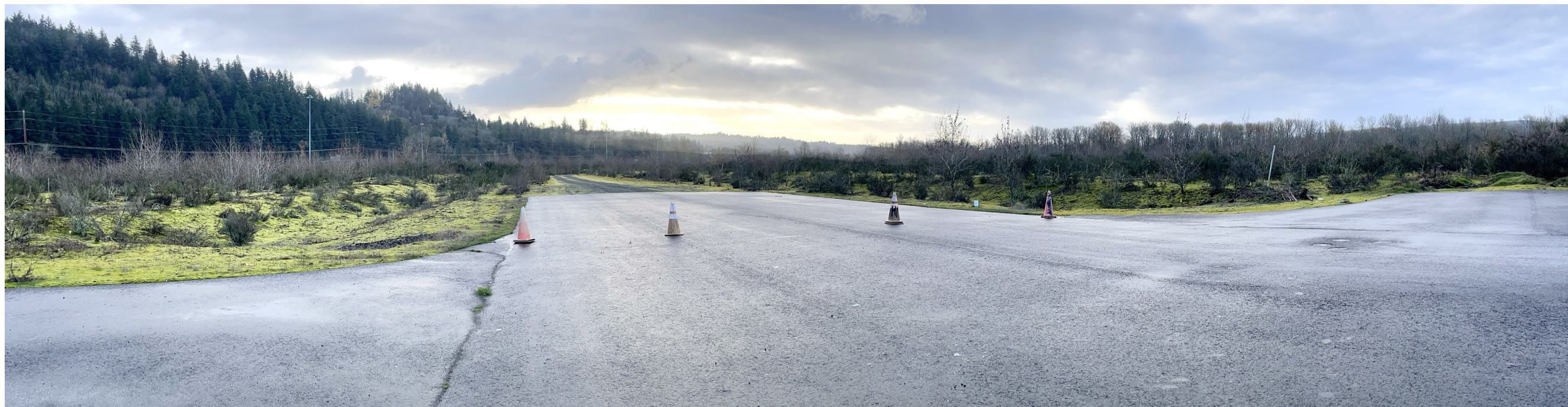
Photo 2: Southern end of Talley Way facing south in the central portion of the study area.
