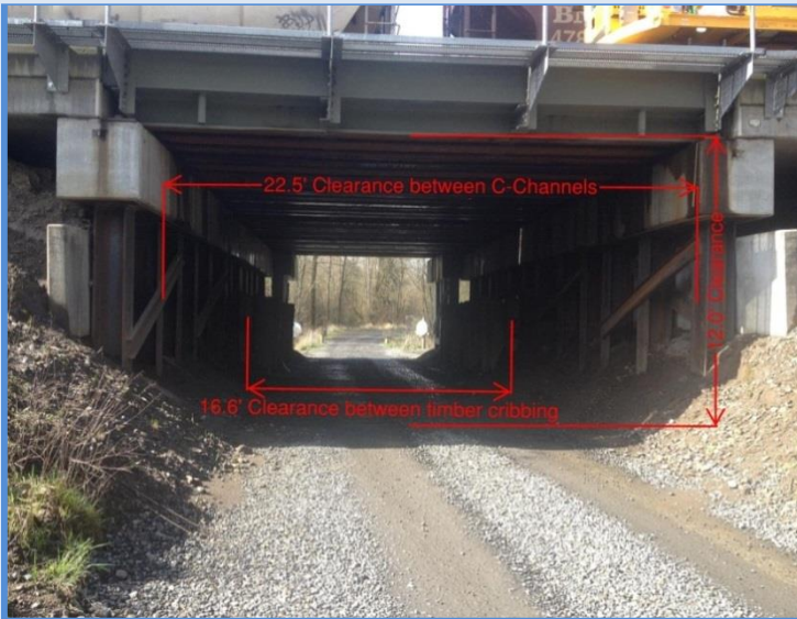
Figure 5: Owl Creek Underpass at BNSF Rail Line
