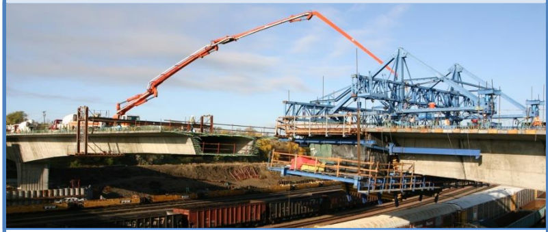
Figure 16: Segmental Concrete Box Girder Bridge Example
