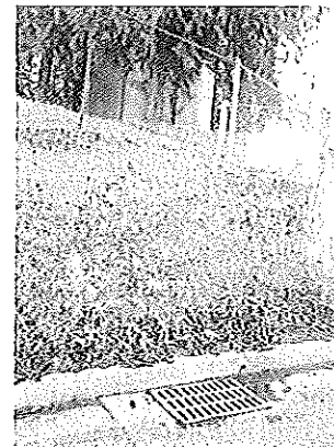
Overview of drain location
