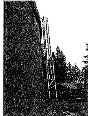
Paxton #2 access ladder
