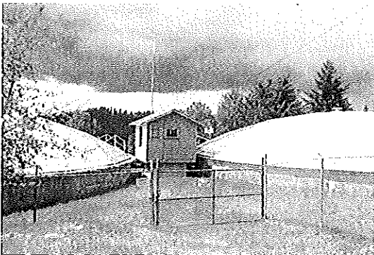
Minor Rd reservoir Bldg in middle houses outlet piping
