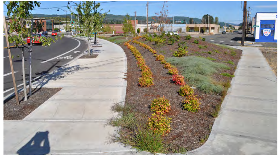
New sidewalks and landscaping along Catlin Street
