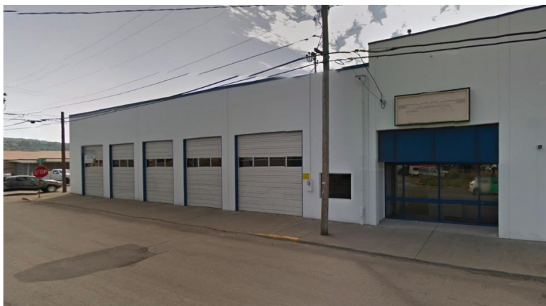
Exhibit 19. Commercial building appropriate for light industrial uses on Catlin St, currently used as a brewery distribution center
