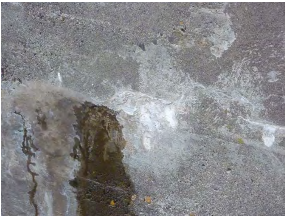
Figure 4: Active Leak, One Of Many (Typical Of Both Reservoirs).
