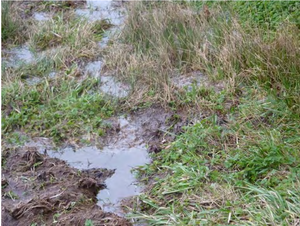
Figure 3: Water At Ground Surface At Downhill Side Of South Reservoir.
