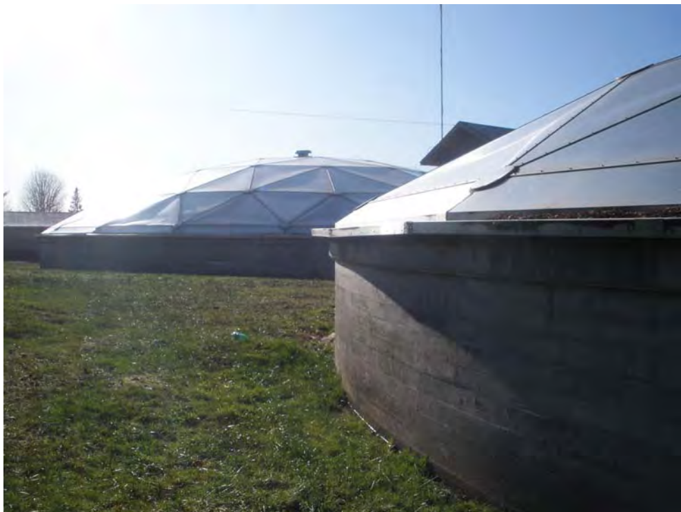
Figure 2: Two Reservoirs At Uphill Side Looking South. Notice The Standing Water Against The Near Reservoir Wall.
