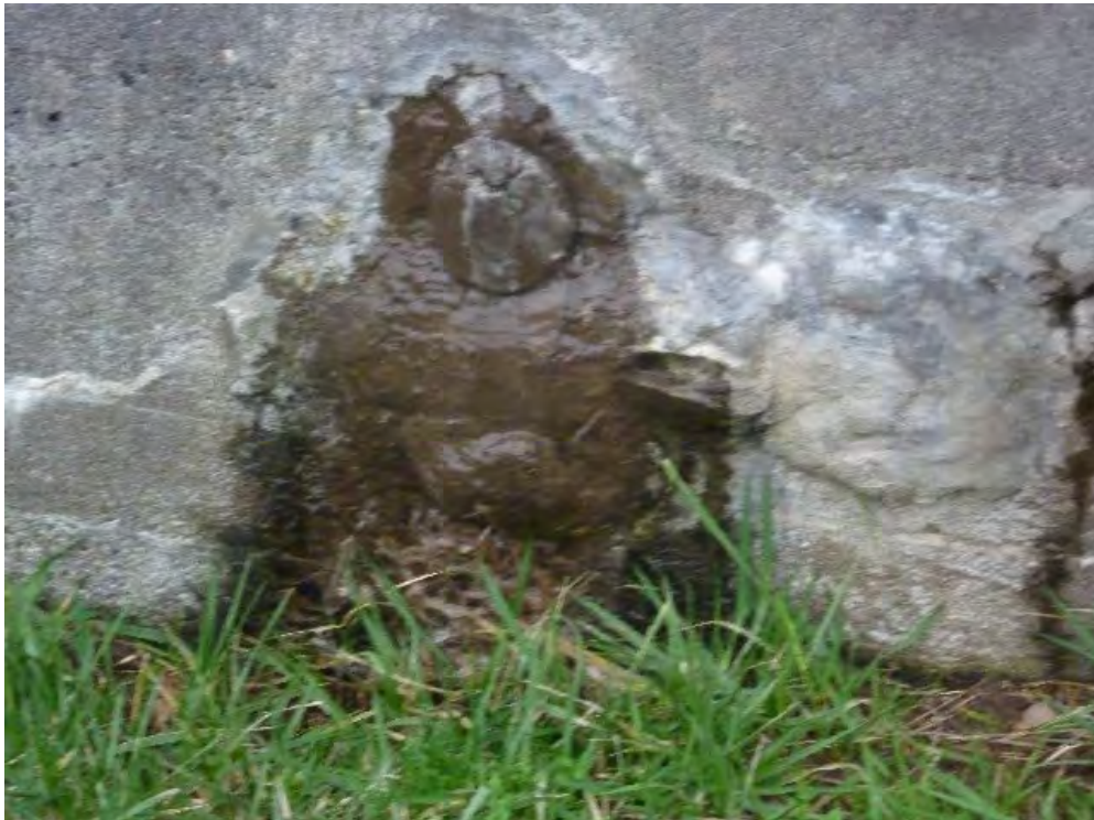
Figure 6: Locations Where Attempts To Patch Leaks Have Not Been Successful.
