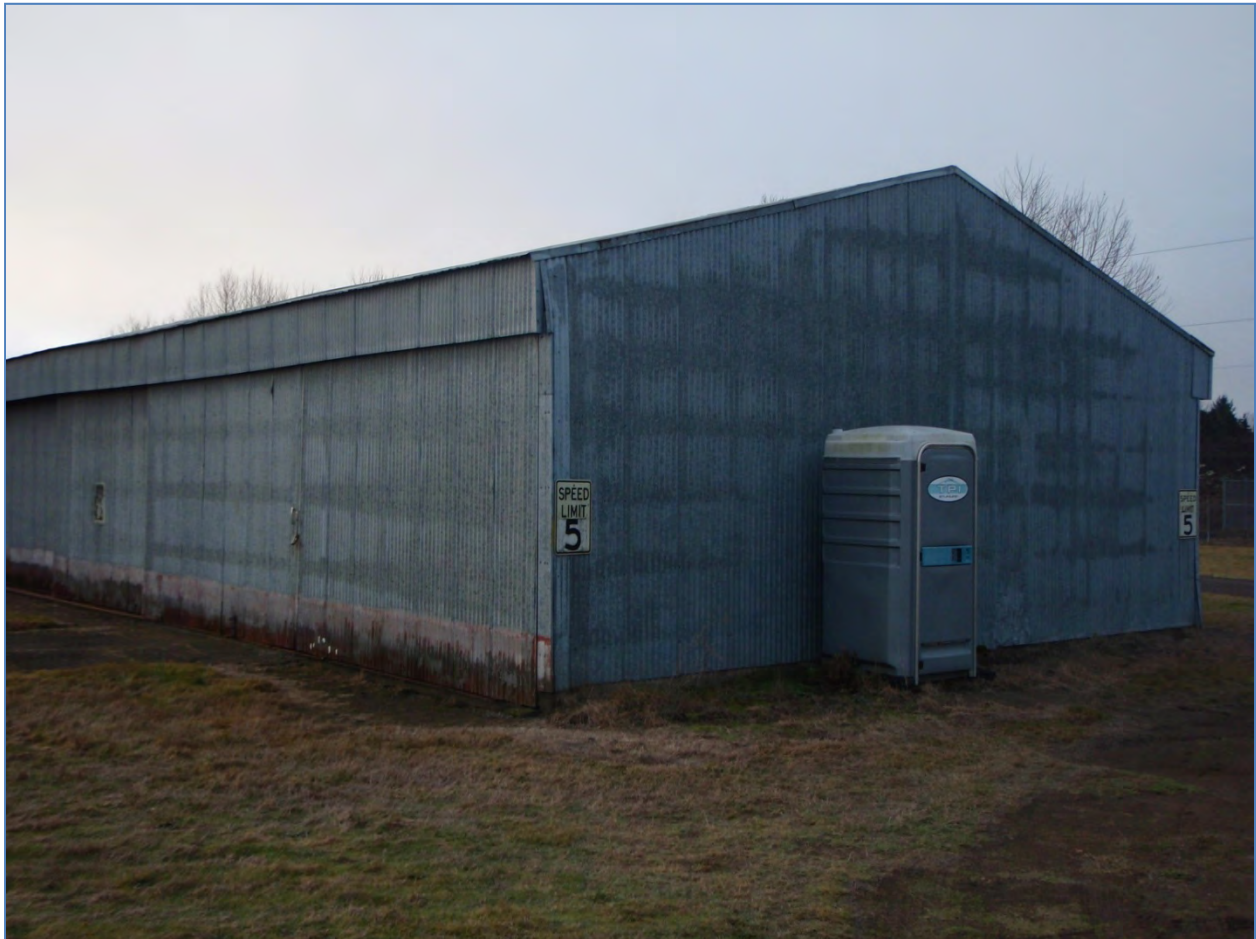
Figure 11. South facing overview of building 15-17/26-27.
