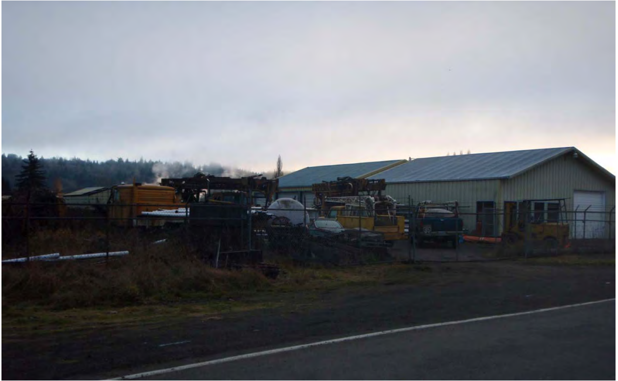
Figure 20. East facing view of parcel 23156 (within fenced area), note metal shop and multiple vehicles.
