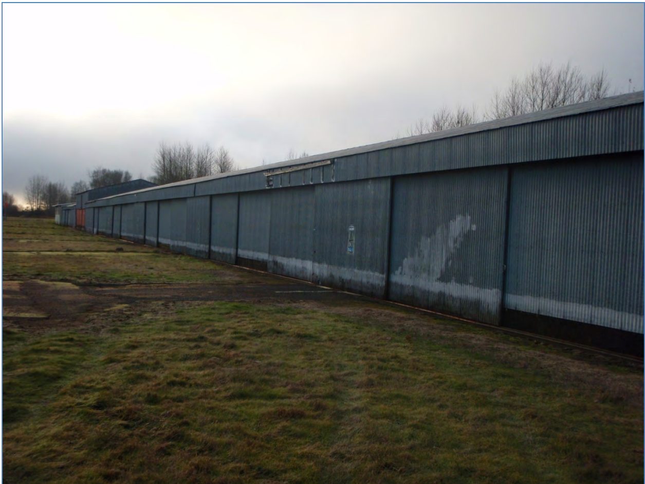
Figure 12. South facing overview of building 18-22/28-32.
