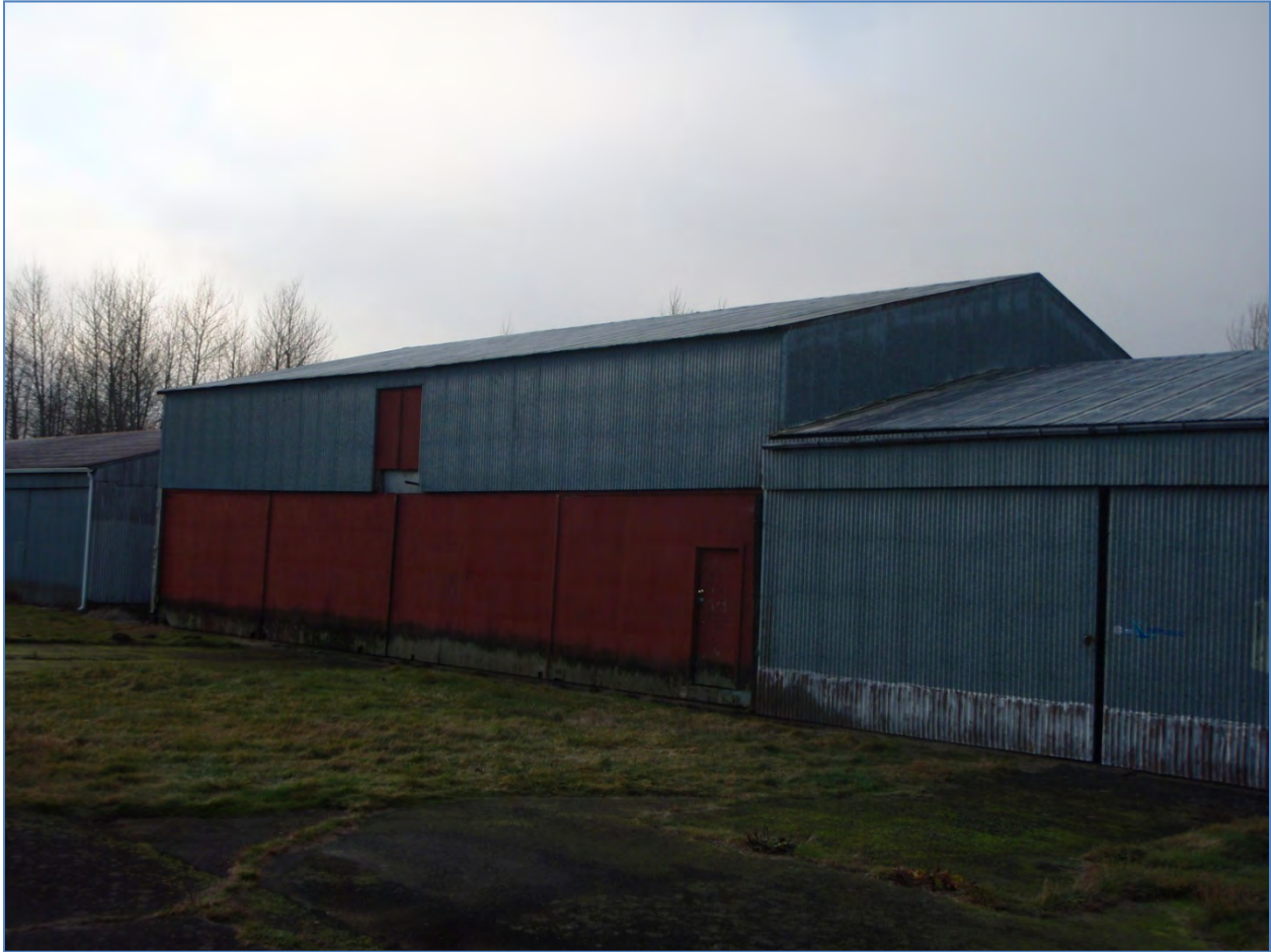
Figure 13. South facing overview of Building 23 (red door).
