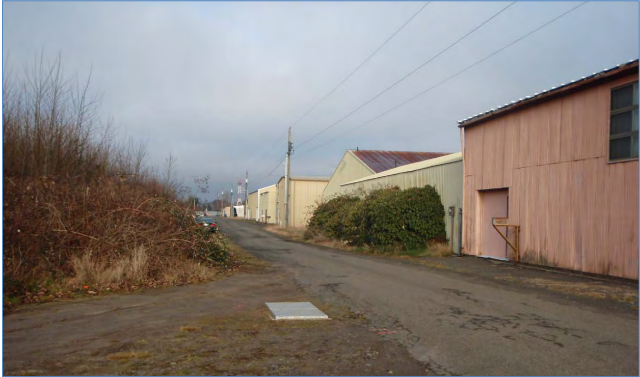
Figure 9. Northwest facing overview of the street side (Pacific Avenue South) of Hangars 35 to 56; note the location of the hangars relative to the street, as well as multiple utility corridors associated with the street and hangars.
