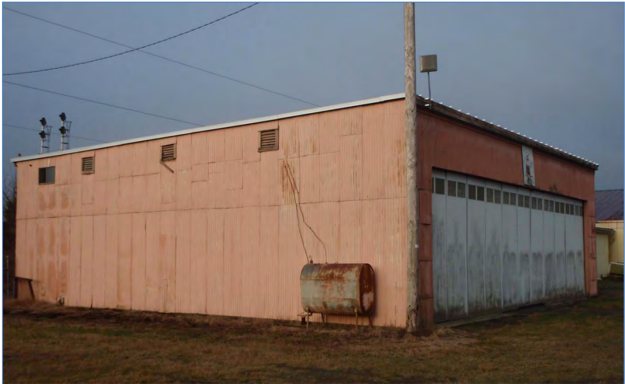
Figure 19. West facing overview of Building 56, recorded as a historic aged hangar structure.
