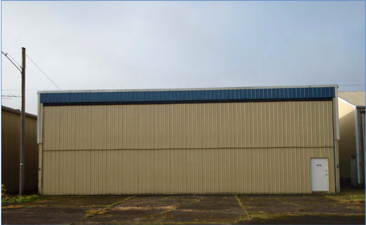
Figure 18. West facing overview of building 48-49, recorded as a historic aged hangar structure (building 48-49).
