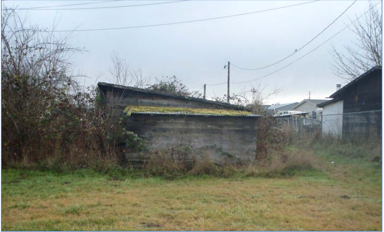
Figure 29. Southeast facing view of shed in the back of parcel 23168.
