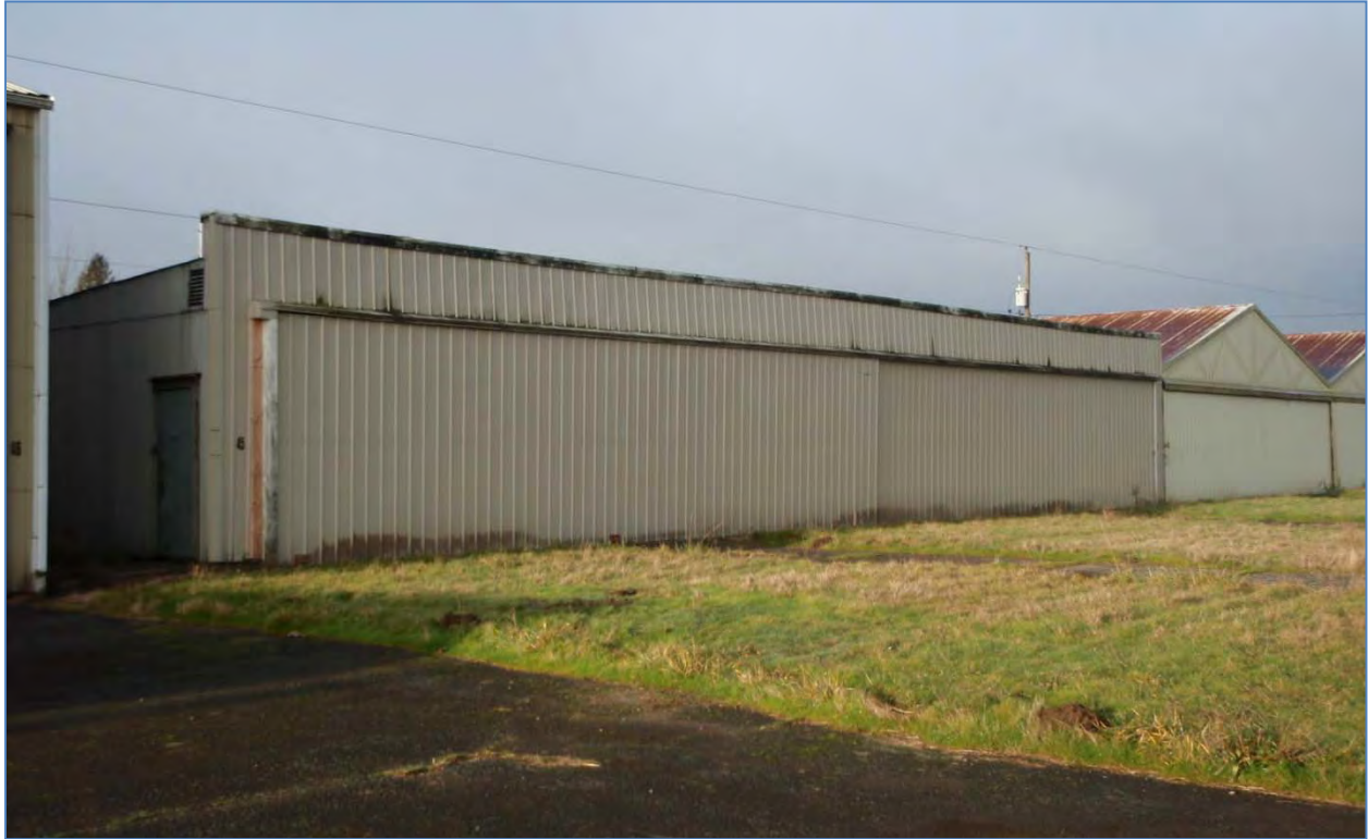
Figure 17. West facing overview of building 44-45, recorded as a historic aged hangar structure (building 44-45).
