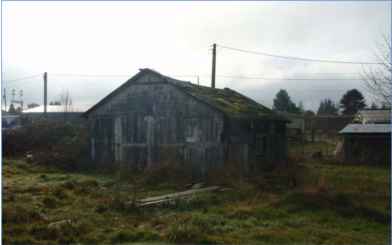
Figure 30. Southwest facing view of the garage in the back corner of parcel 23168.
