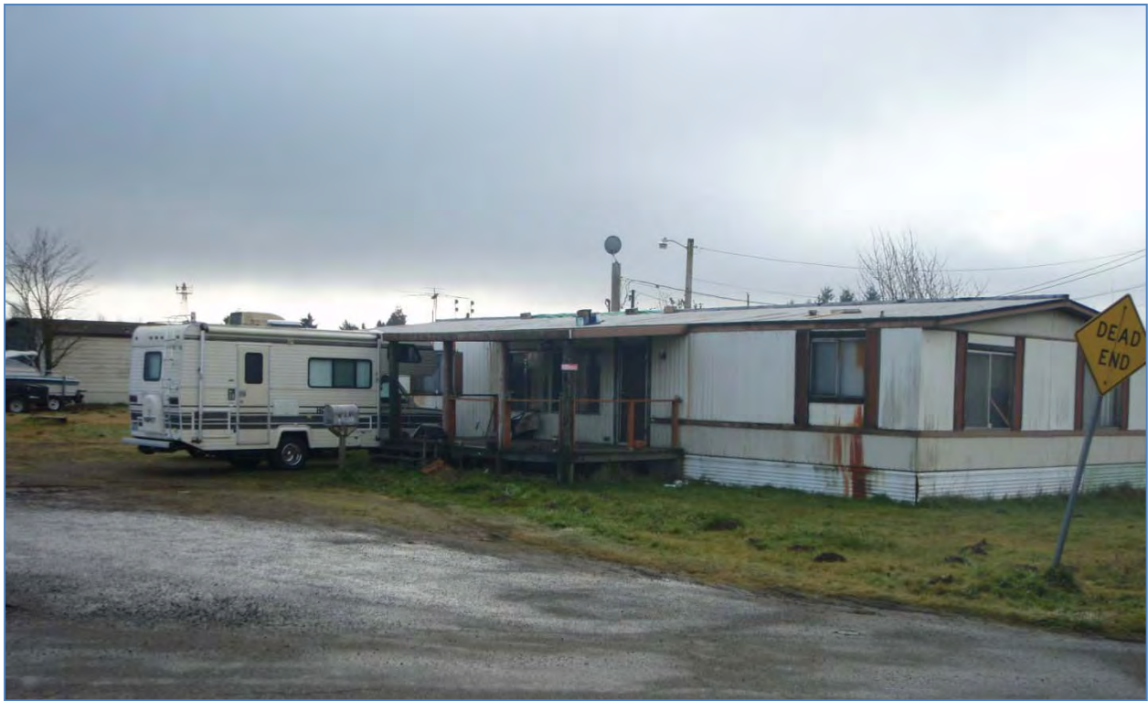
Figure 28. South facing view of building on parcel 23168.
