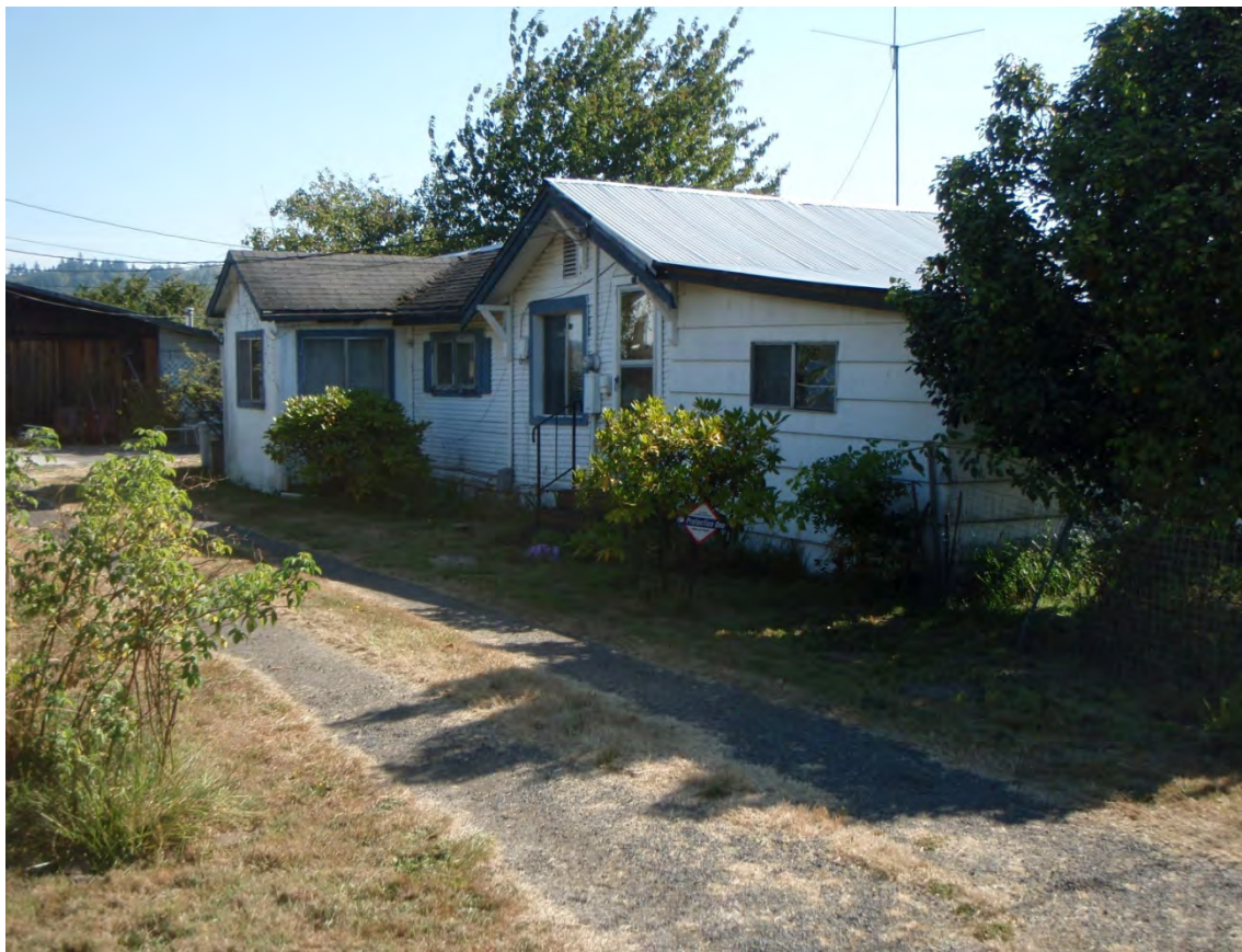
Figure 22. North facing view of the single story house and garage (brown structure on left edge of frame) at 23158.
