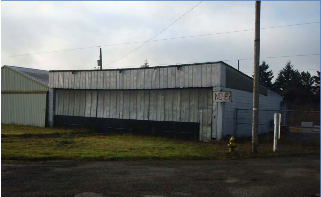
Figure 16. South facing overview of building 41, recorded as a historic aged hangar structure (building 41).
