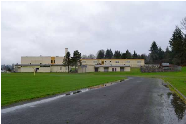
South elevation, field house, wood shop, and athletic field overview, facing north
