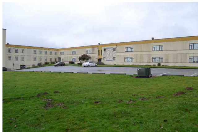
South and east elevations and parking lot, facing northwest
