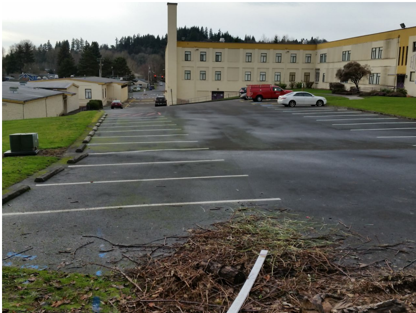
Photo 3. Areas immediately adjacent to the school buildings have been landscaped and contain underground utilities. The view is towards the west.
