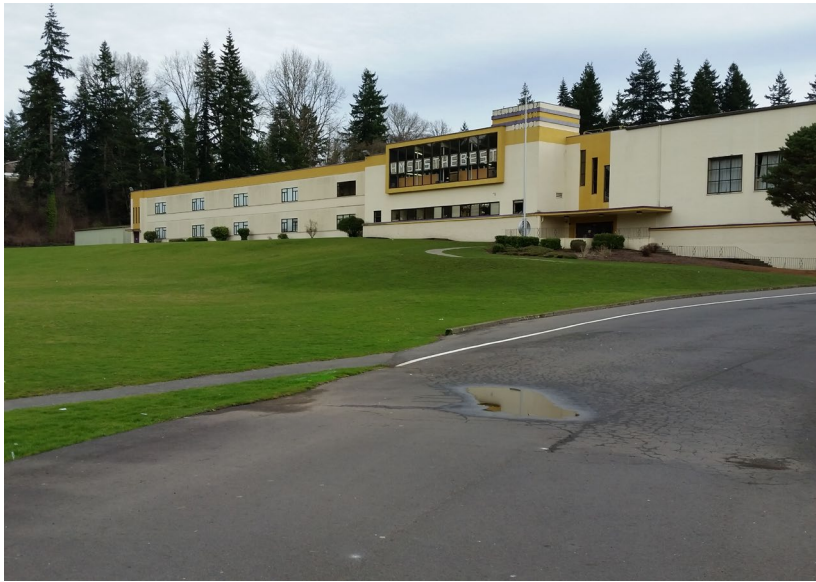
Photo 1. Huntington Middle School is constructed on a fill platform above the natural landform. The main parking lot is in the foreground at right (southwest). The view is towards the southeast.
