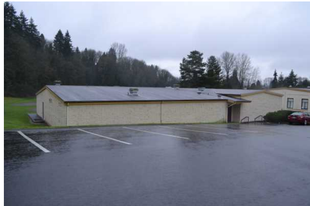
Field house north and east elevations, facing southwest
