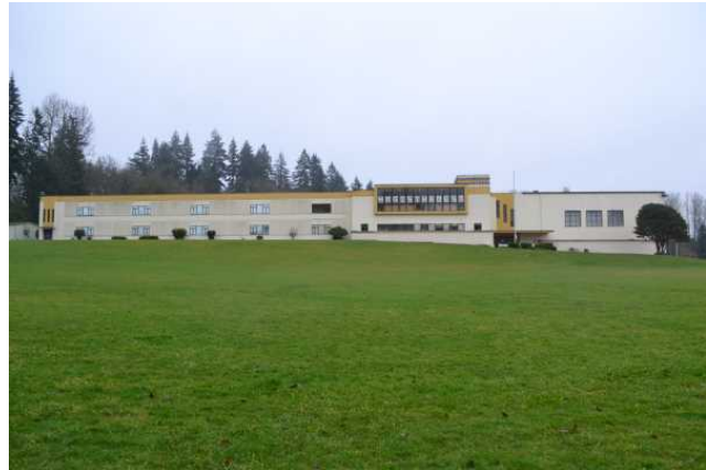
North facade, facing south
