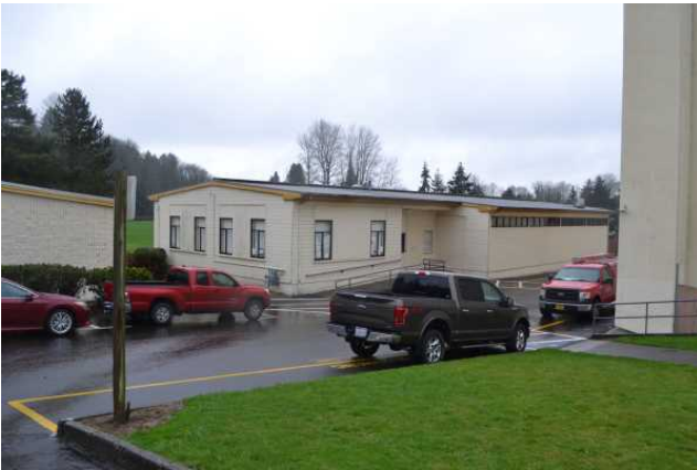
Wood shop north (primary) and east elevations, facing southwest
