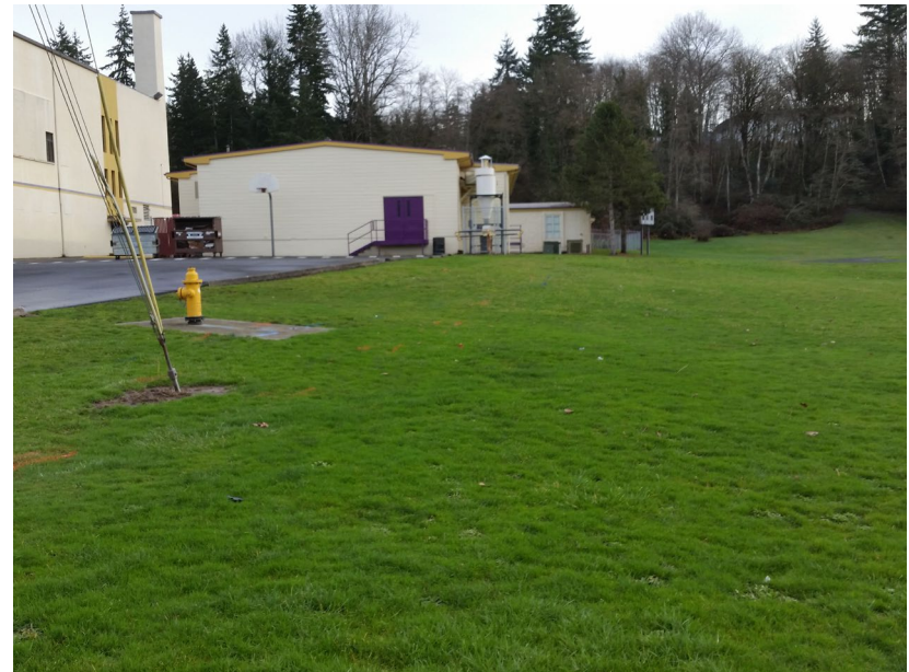
Photo 4. Underground utilities extend throughout the base of the fill platform south of the school. The view is towards the east.
