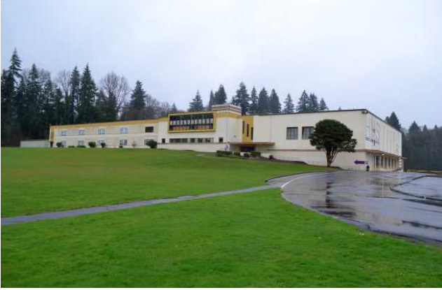
North (primary) and west elevations, facing southeast
