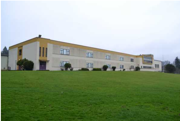
North (primary) and east elevations, facing southwest
