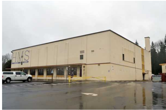
South and west elevations of cafeteria/gym wing, facing northeast
